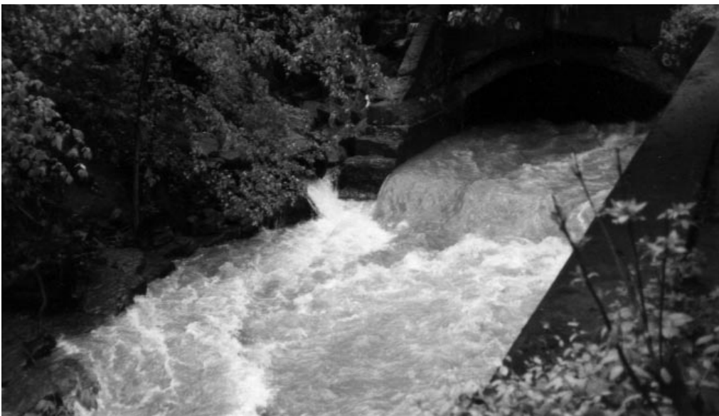
The Wilkinsburg culvert after rainfall
