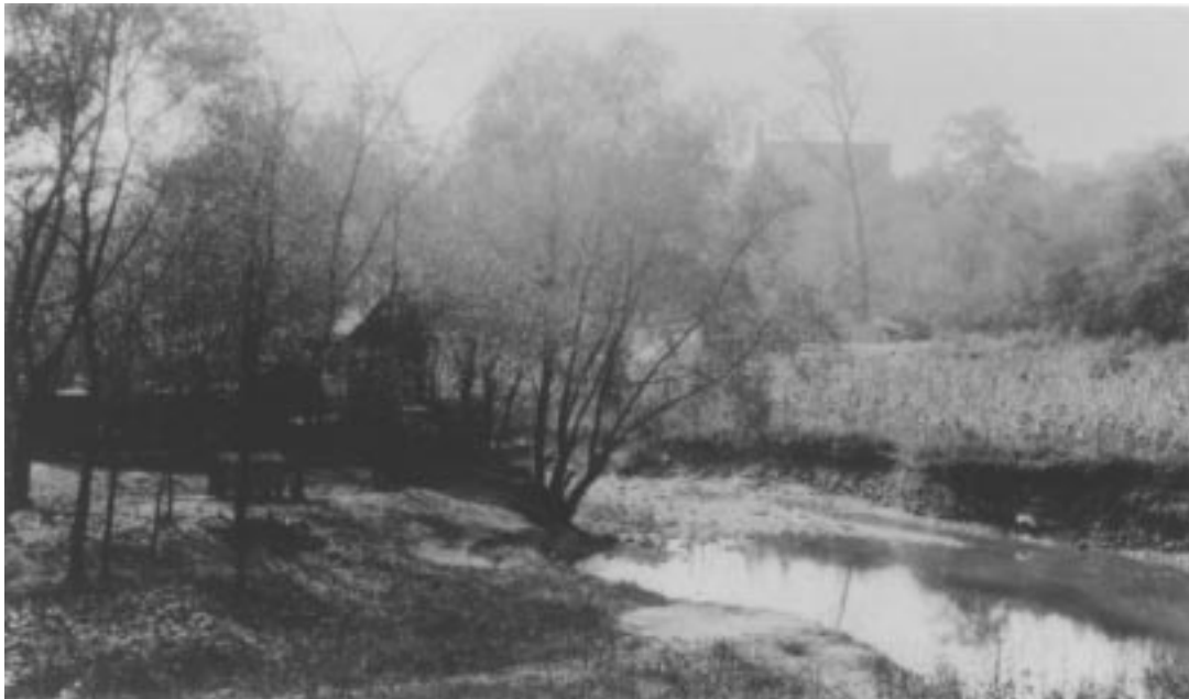
A view of Nine Mile Run just before construction of a culvert circa, 1923. This section of the stream presently lies under Greendale Avenue in Edgewood. Photo courtesy of Ted Rakovsky
