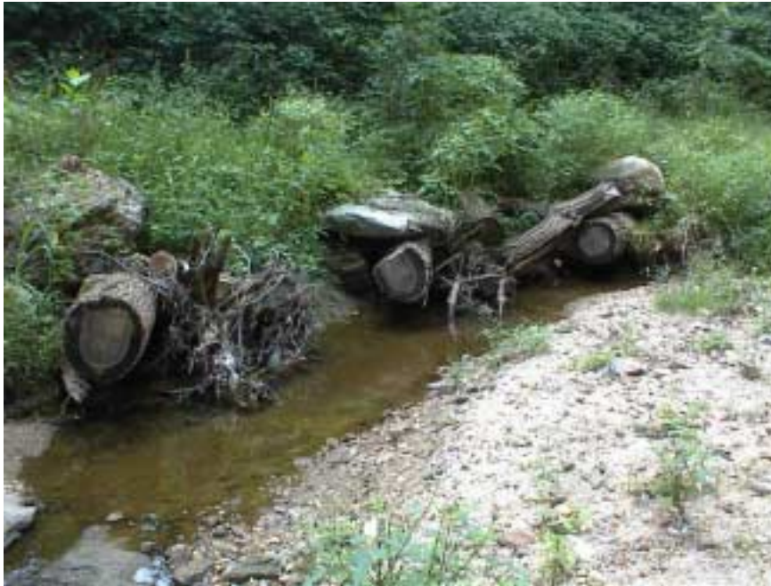
Figure 5.4.1: Root Wad Channel Stabilization
