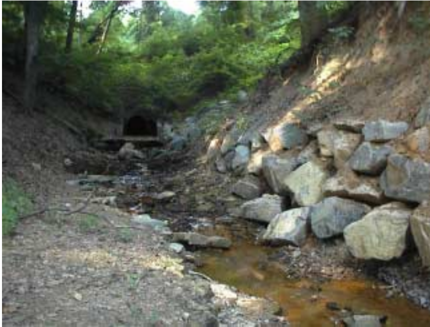
Figure 5.4.6: Typical Example of Boulder Bank Stabilization
