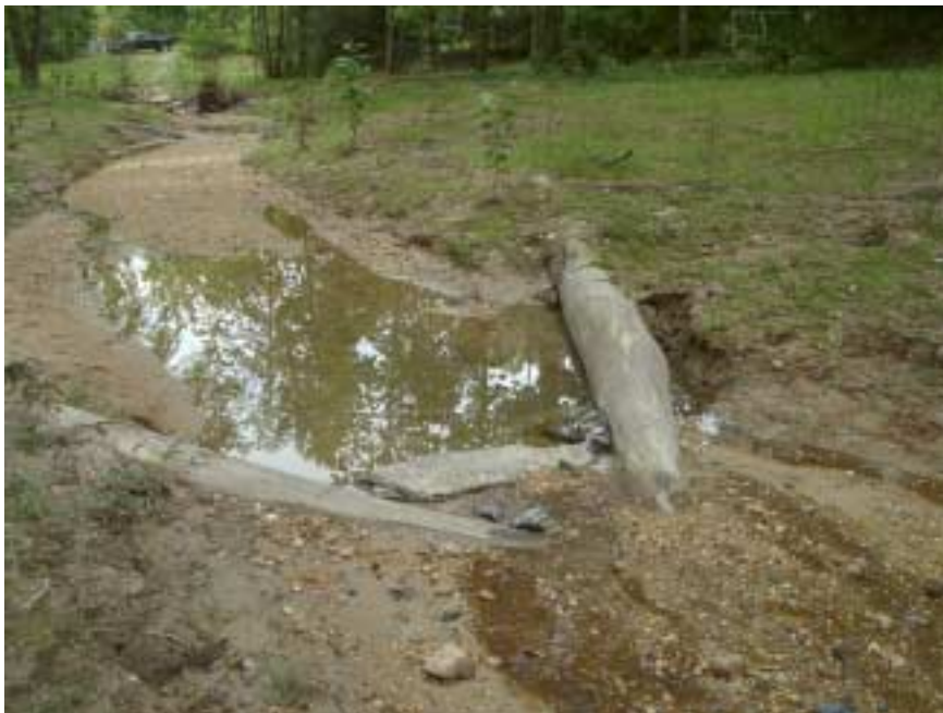
Figure 5.4.2: Typical Example of a Log Vane
