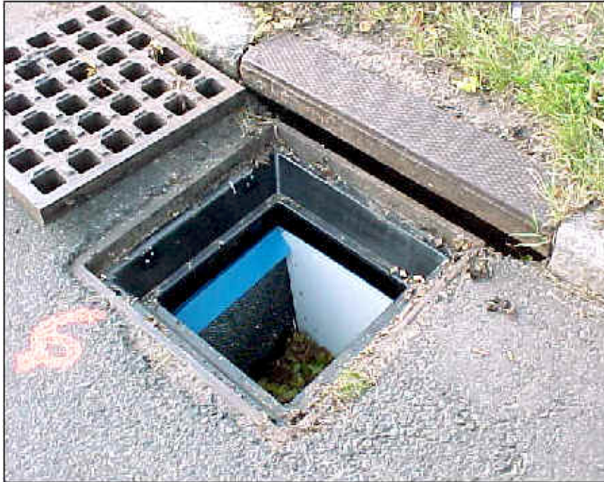
Figure 5.2.5: Typical Storm Inlet Filter
