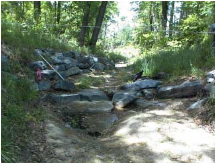
Figure 5.4.4: Typical Rock Cross Vane
