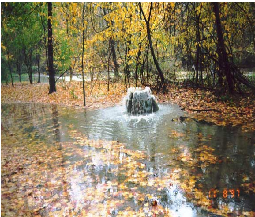
Figure 4.3.9: Sanitary Sewer Overflow in NMR
