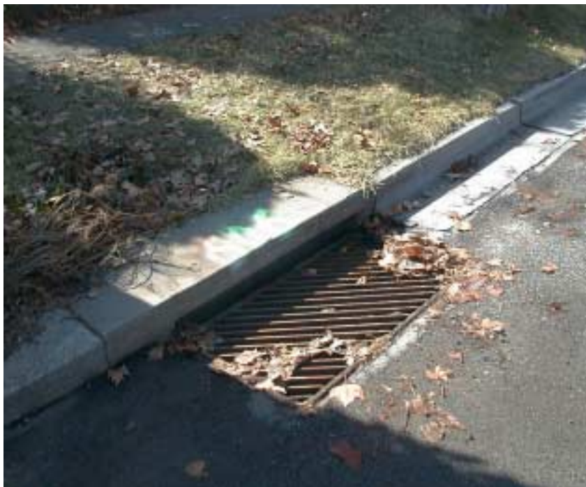
Figure 4.3.4 Typical Storm Inlet in NMR
