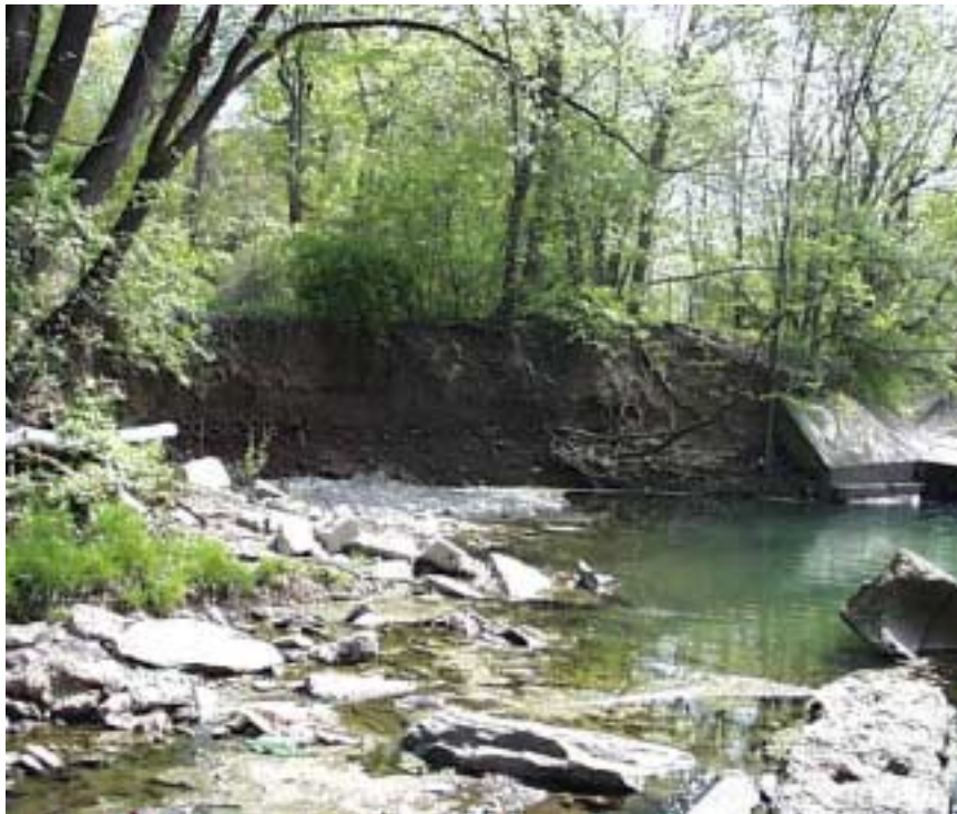
Figure 4.1.3: Channel Erosion of NMR Stream
